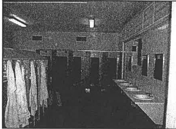
Housing Toilet Room Upgrade
